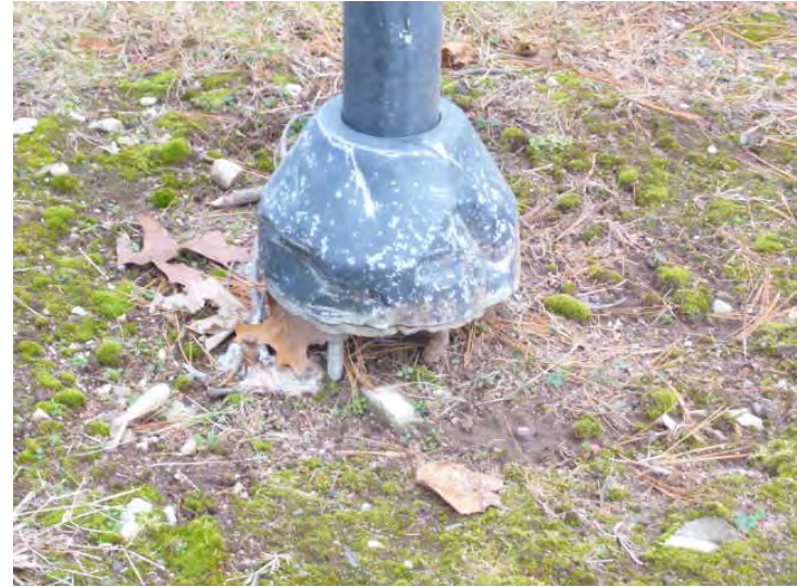
Original site light fixture footings and light poles are in poor condition. New heads have been installed.
