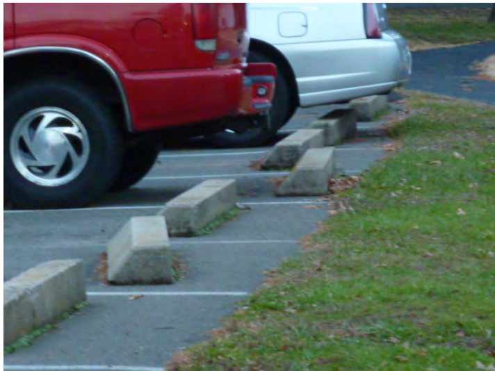
Concrete parking bumpers should be re-pinned.
