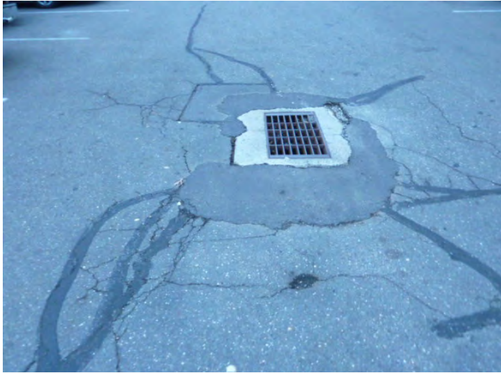
Crackfill and sealcoating is needed at asphalt drives and parking.
