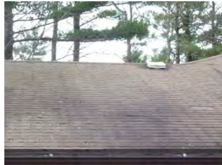
Asphalt roofing deformed and missing shingles at E-40.
