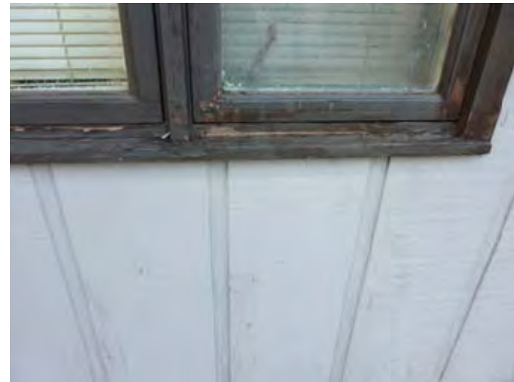
Typical wood windows at E-82 are in poor condition.
