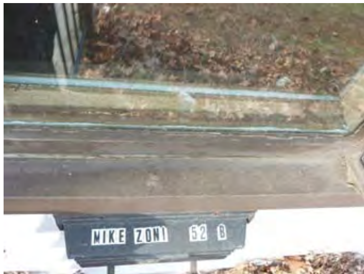
Windows at E-40 are typically original single glazed wood units in poor condition.
